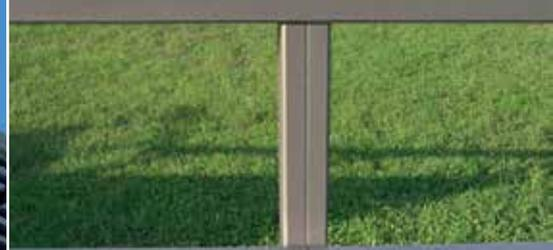
Long façades: Railing segments are coupled together with two half posts, which provide a seamless transition on long façades.
