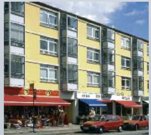
With an enclosed balcony, heat gain through passive energy is the result of a greater window to floor ratio than that of an open balcony or traditional window. **Sustainability**, thus heat retention, saves energy and money, whilst frameless panes maximise natural light; and reduce energy requirement. Natural ventilation eradicates the need for expensive and energy consuming air conditioning/moisture extraction equipment.
