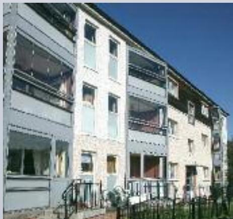
Enclosed balconies, as part of your renovation programme, can be fixed to the existing fabric of your building. This means that the glazing is able to protect the buildings façade resulting in lower **maintenance costs** arising from dirt and general wear and tear.
