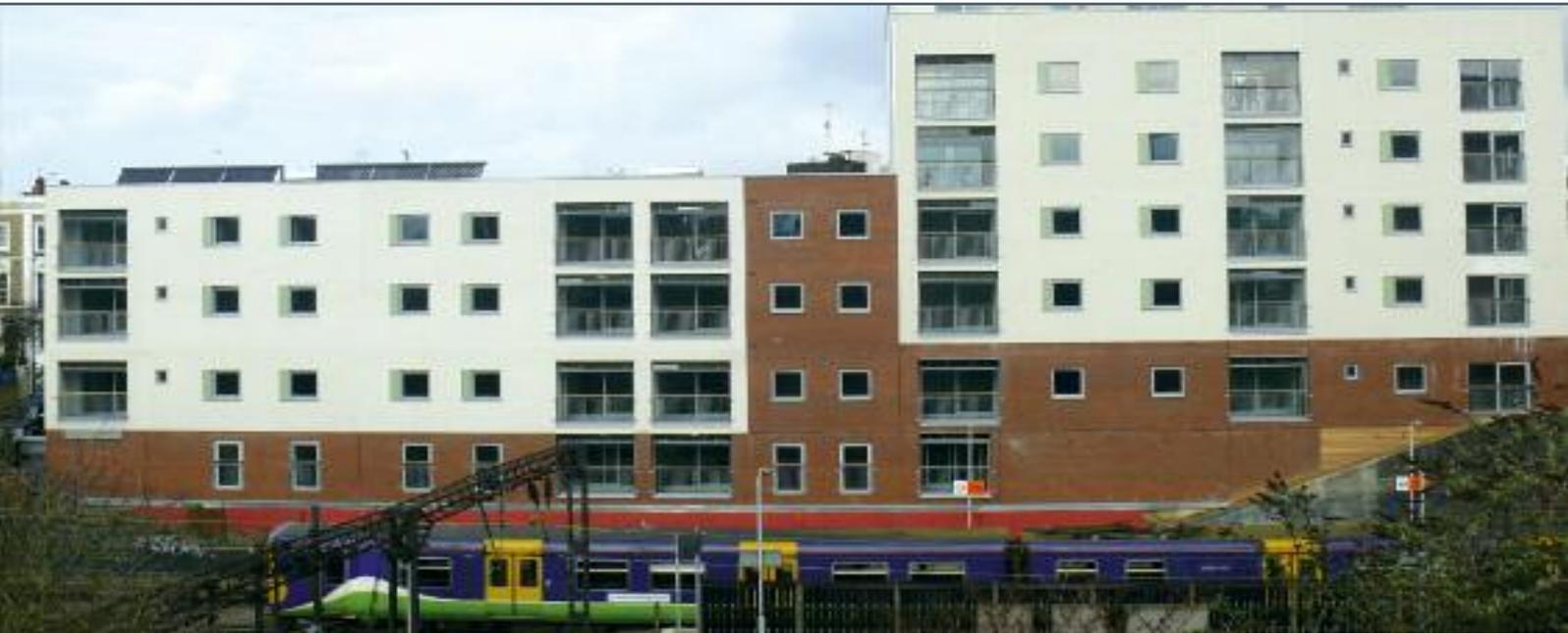
"The Belsize Road development was built on a tight site, immediately adjacent to the main line into Euston station. Many of the flats had balconies overlooking the line, and we wished to provide a screen that would shelter the space from the noise of the trains and prevent objects from falling onto the line below, while providing suitable levels of ventilation and daylight. Windoor designed a lockable screen that satisfied both Railtrack and our Client, Notting Hill Housing Trust."
